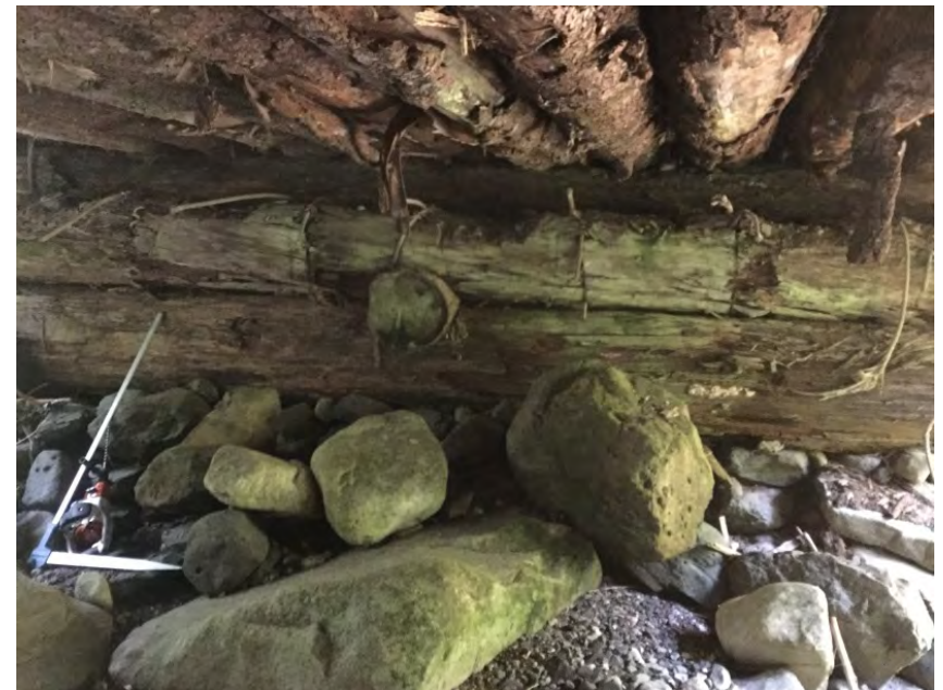
Left Bank Abutment when facing downstream
