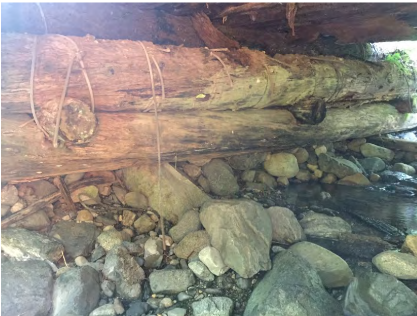
Right Bank Abutment when facing downstream
